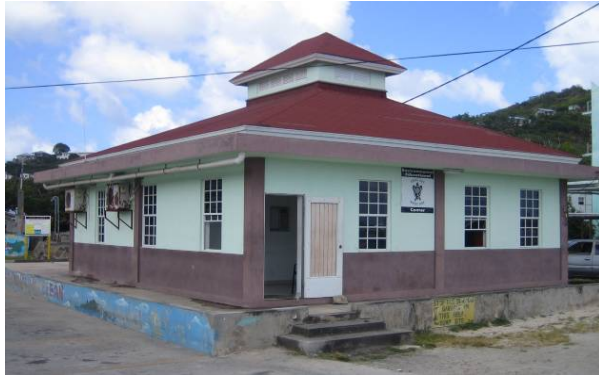
Figure 13. The new TCMP office in Clifton, Union Island.
